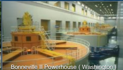
Bonneville II Powerhouse ( Washington )
