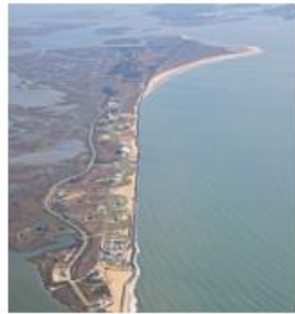
Seawalls and Revetments
