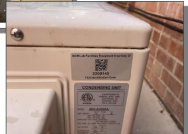
Administration Building / Observatories / D305006.4 / 1
