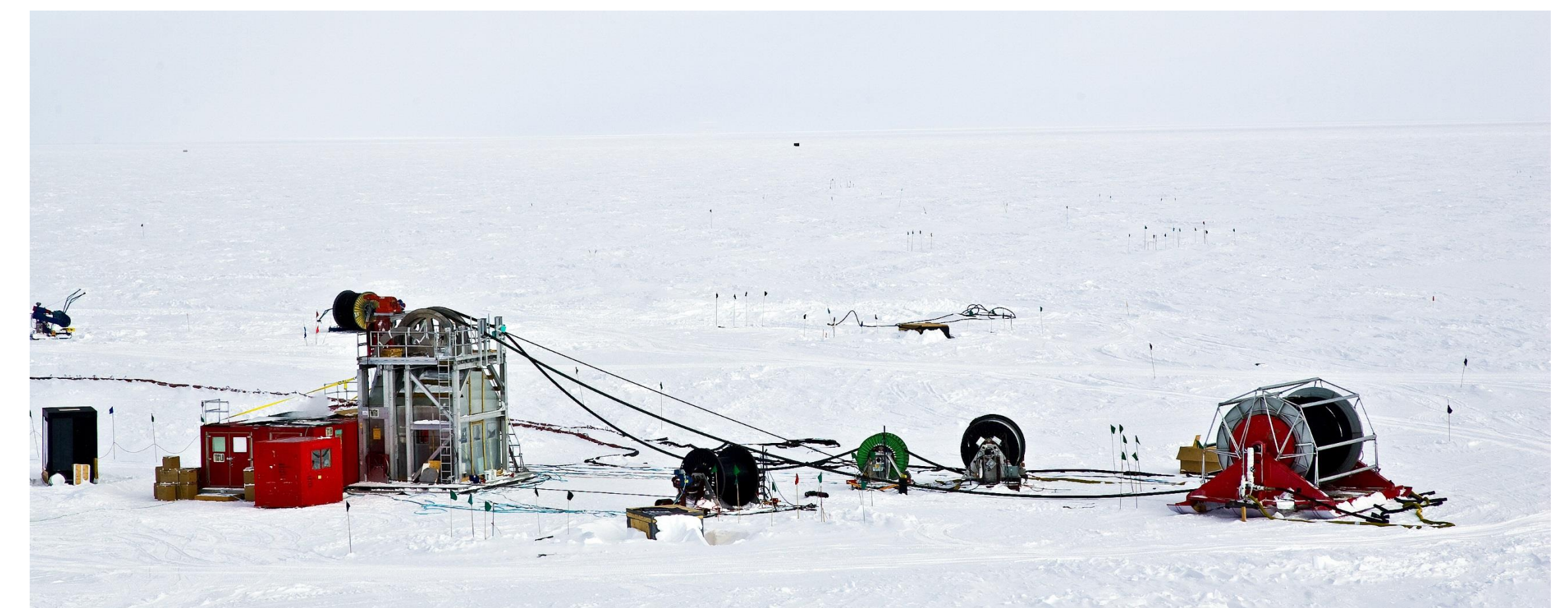
Tower Operations Site, top of borehole is inside tower structure
