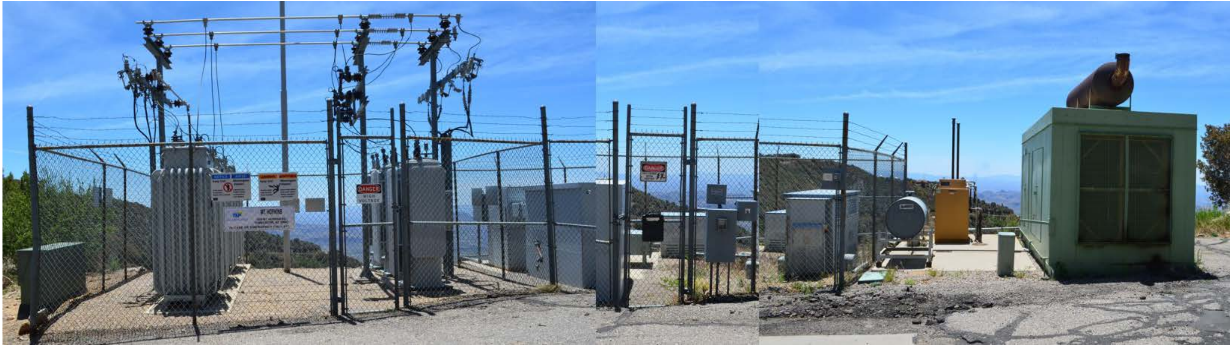
Existing Unisource Power 13800v Substation
